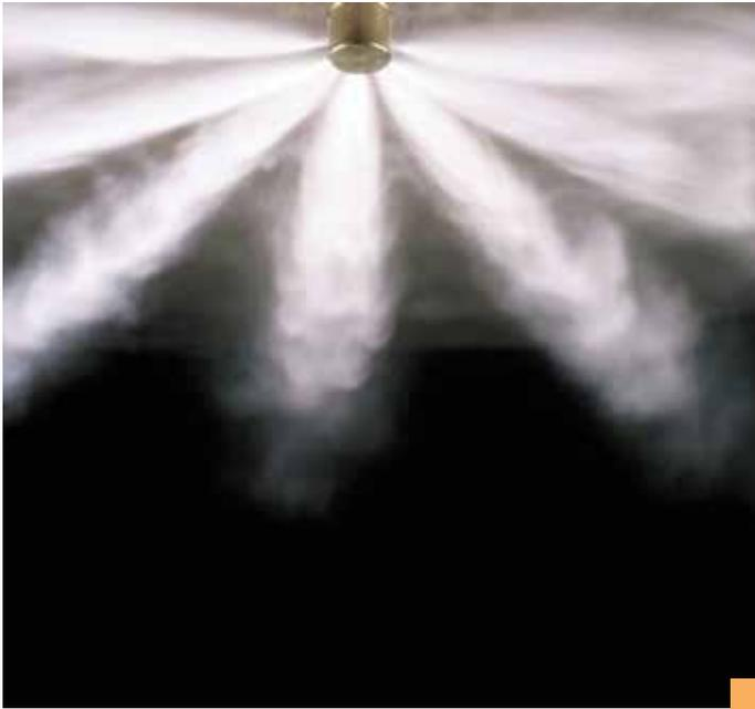
*VSN 1230 fire extinguishing systems fight fires using Novec™ 1230 by 3M™. This extinguishing agent is particularly suitable for the protection of spaces with electronic and electrical equipment and offers an economical fire protection solution especially for small and medium-sized rooms. The 50 bar technology of the VSN 1230 system makes optimal use of the characteristics of this extinguishing agent.*
